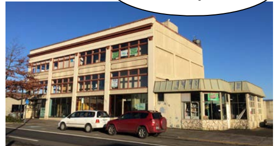
1210 Marine South Façade
